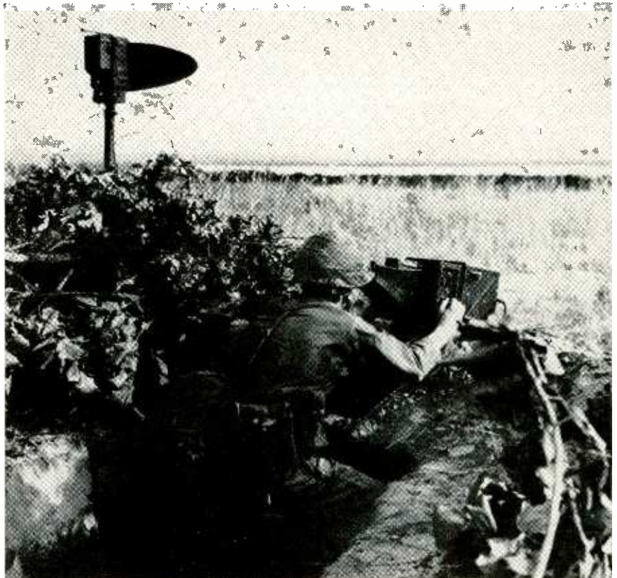
The remotely operated AN/PPS-5 is scheduled to replace the PPS-4 as the Army's front line surveillance radar.
